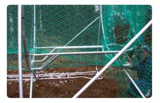
**15.** Make sure that the box holder is centered. Drill a hole through the pre-drilled holes of the box holder and through the centre of the ring.
