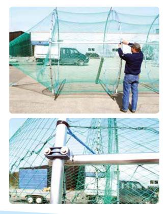
**4.** Attach the aluminium benders (4 pcs) on one side. The longest tube on the bender should be attached to the upper bracket.
